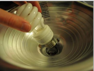
Locate the bad bulb and remove it from the socket. This is achieved by grabbing the bulb lightly and rotating counter-clockwise.
