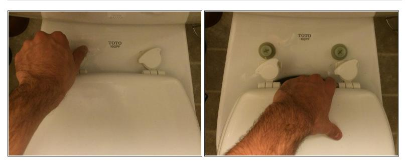
Twist the tops of the hinges of the currently installed toilet seat and pull toilet seat off to expose the screws.
