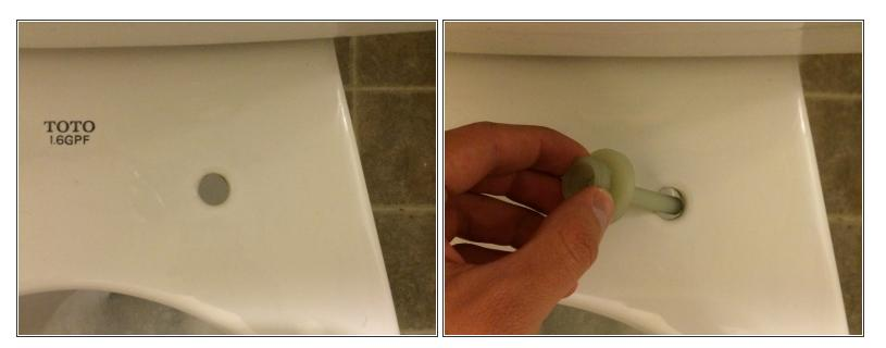
Insert new special 20mm screws that are provided with the purchase of the toilet seat in the holes and tighten them.
