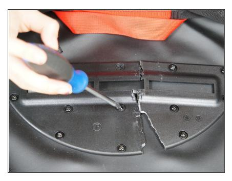
While holding nuts with the wrench, use the screwdriver to unscrew the screw in the front bracket.
