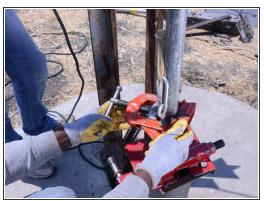
Attach and tighten the elevator clamp to the riser main as close to the bottom as possible.
