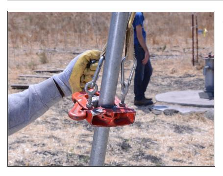
Remove the elevator clamp from the riser main, and secure it to the tripod to keep it out of the way.
