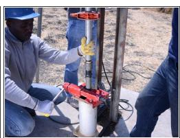
• Once the first joint is exposed, tighten the base clamp below the joint.
