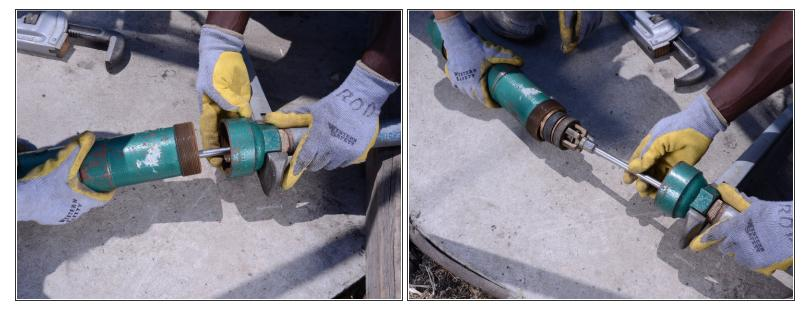
• Slowly pull the cylinder off of the pump rod, exposing the traveling valve and foot valve.
