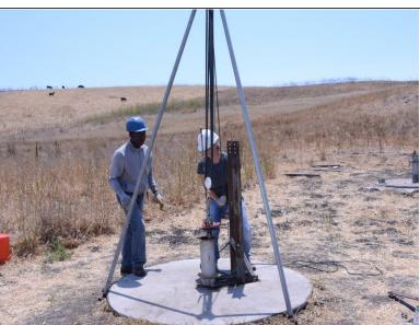
Being careful not to let the rope slip, use the block and tackle to lift the riser main until the pipe elevator reaches the block and tackle.
