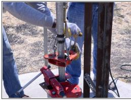
Remove the clamp from the riser main, and repeat steps 23-25 until first joint is exposed.
