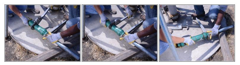
Using two pipe wrenches, unscrew the cylinder from the riser main.
