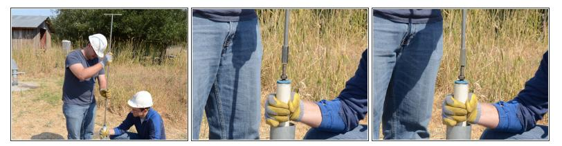
• Screw the T-handle onto the top of the riser main.
