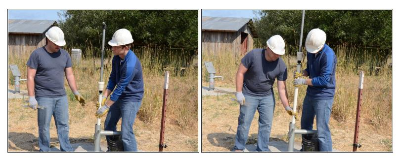
Lift up the handle and riser main until the joint between the two is at a comfortable height to work on.
