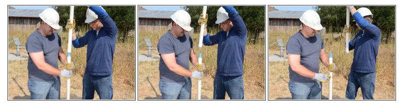
• Remove the top section of the riser main.
