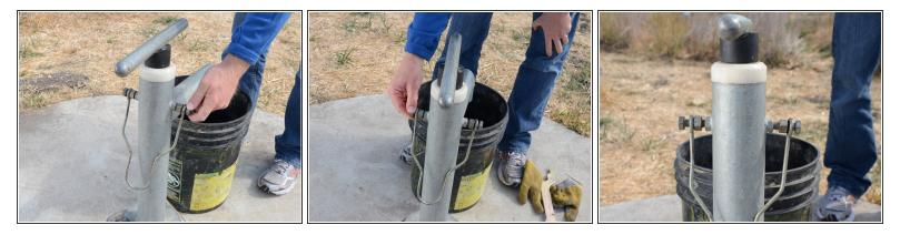
• Unscrew the lock bolts about half an inch.
