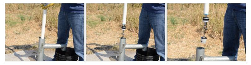
(i) The last section of riser main will have the traveling valve screwed on to the end, and the foot valve hooked onto the traveling valve.
