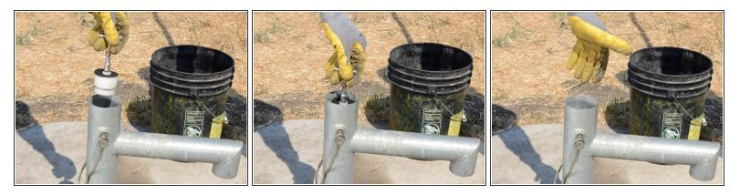
When reassembling the pump, drop the foot valve down the well in the proper orientation, and follow the directions in reverse.
