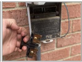
↑ Turn off the power before beginning by pulling the plug or flipping the switch on the disconnect box. Leaving the power on during the repair could result in death or serious injury.
