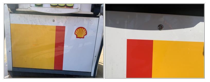
After the filter has been installed, reattach the panel cover and lock it in place.
