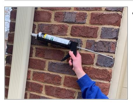
Apply the silicone caulk to the joint area to seal leaks and reassemble the gutter system.
