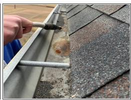
Clean the area around the leak with a wire bush or garden trowel and a bucket, taking out the leaves and debris placing what you remove in the bucket and flushing the gutters with water using a hose to make sure you have a clean area, as well as rinsing and drying the area thoroughly.
