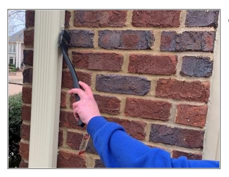
Clean any caulks from around the downspout joints using a stiff wire brush.
