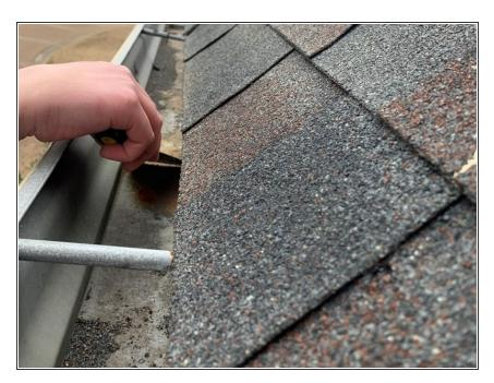
Smooth out the cement by using the putty knife or trowel so that can smooth out any rough edges.
