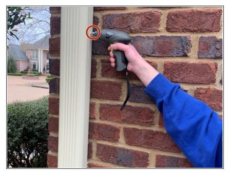
Remove any screws or connecting hardware at the joint of any leaking or worn portion of the downspout and then disassemble any leaking or worn portion of the downspout joint.
