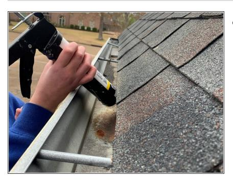
Apply plastic roofing cement to any holes present in the gutters by working it into the hole or crack with a putty knife or trowel.
