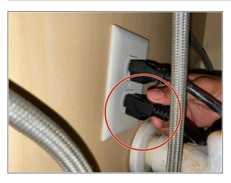
Install and plug electrical wire into the correct power source. Test your disposal switch and check for any signs of leakage.
