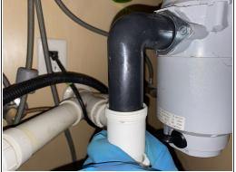
After mounting the disposal in place, align the black disposal pipe with the white PVC pipe connected to the sink.
