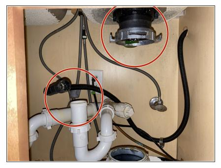
Before installing your garbage disposal, make sure both your pipes and garbage disposal mount (pictured at the top) are aligned correctly to support your model.
