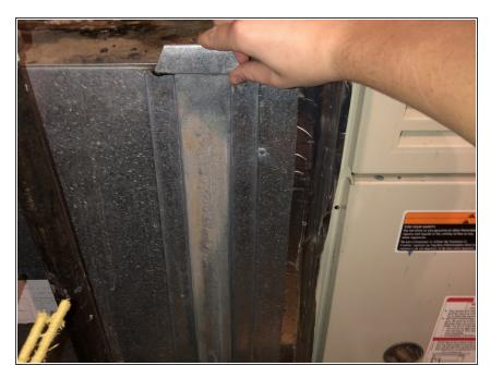
• Close the door to the filter and make sure it is snug with no air leakage.
