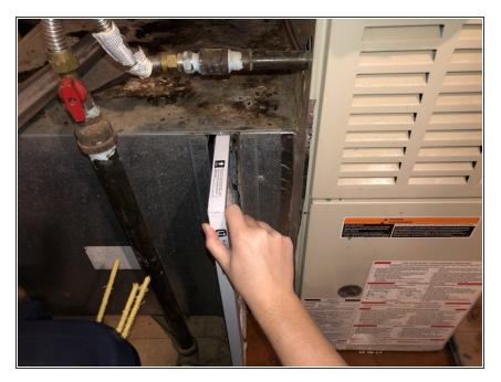
Place the new filter in the unit with the arrow pointing towards the air conditioner unit.
