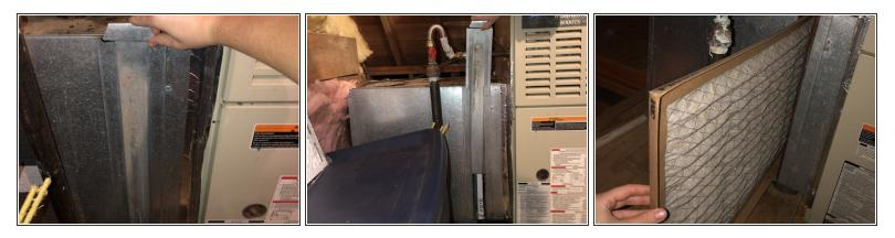
• Open the filter access door and pull the old filter out.
