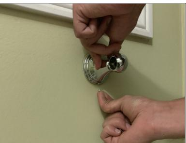
Insert the screws into the holes beneath each bar holder.
