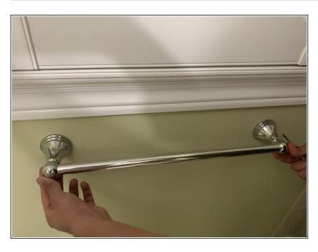
Place the new towel bar on top of the wall brackets and make sure that the bar is level.
