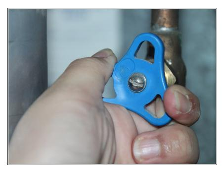
Turn the water shutoff valve counterclockwise to the "off" position.
