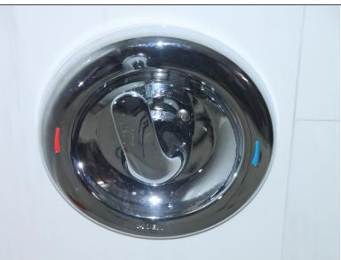
Turn the handle of the shower valve 180 degrees until it is in the "up" or "on" position.
