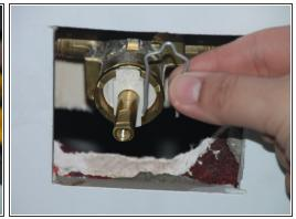
• Slide the tip of needle-nose pliers under the notch of the retaining clip and pull the clip upwards.
