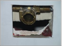
Clamp firmly onto the brass tube with a pair of vice grips and gently but firmly pull out the cartridge.
