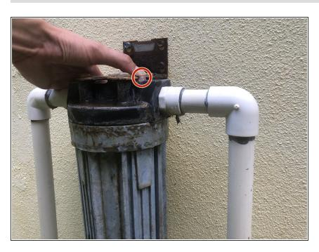
Press the button on the top of the device to release any air trapped inside.
