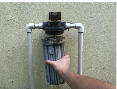
Unscrew the filter canister using the canister wrench.
