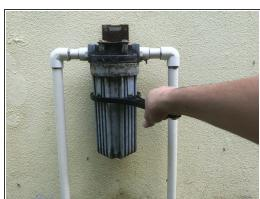
Screw the filter canister back into place using the canister wrench, making sure it's tightly screwed
