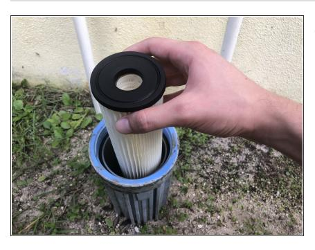
Put the new filter inside the filter canister, making sure it goes in properly.
