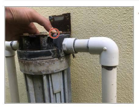
Press the button on the top of the filtration device to release water pressure and let excess water drain.
