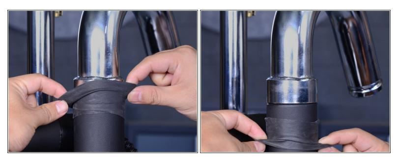
• Peel the rubber sleeve down from the elbow pipe to reveal the pipe socket.
