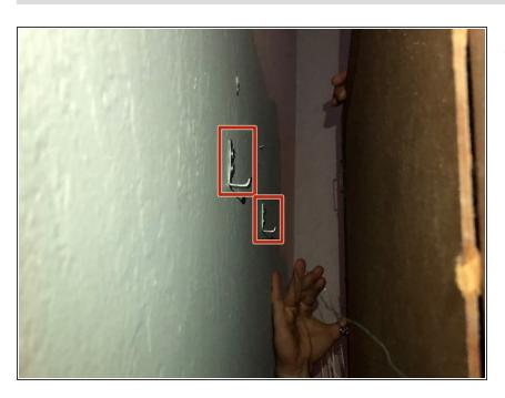
Align the mirror to the center of the metal anchor and hook the wire on.
