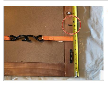
Measure 14 inches down from the top of the mirror to place the screw and loop found in the anchor kit.
