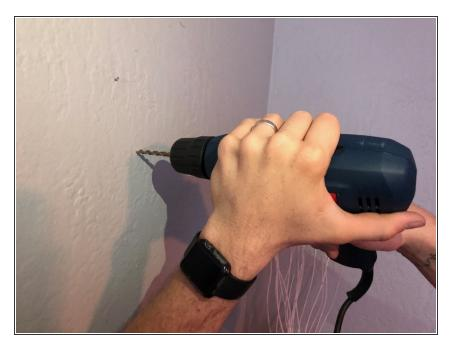
Drill one hole in the wall, and about 1/2" underneath that hole, drill another hole. It should be the same size and distance as the metal anchors.
