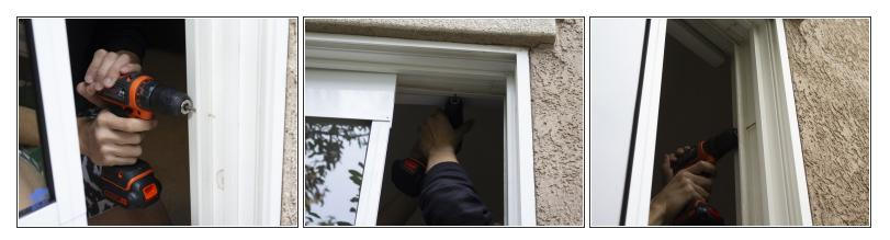
With a <u>9/64ths drill bit</u>, drill clearance holes into the marks made on the sliding glass door frame
