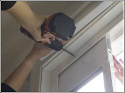
Repeat steps 8 and 9 to secure the dog panel into place. Follow these steps when drilling into the clearance hole marked at the top of the frame.
