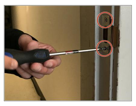
Screw in the top screw first, ensuring that the strike plate will remain in place. Then, screw in the bottom screw.
