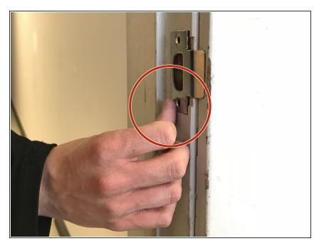
Apply the new strike plate to the frame of the door, and ensure that the strike plate's holes are aligned with the drilled-in holes on the door frame.
